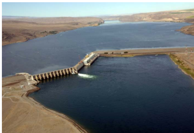
Figure 8-7. Large hydroelectric plant
