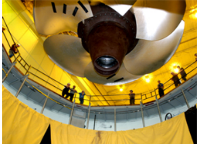
Figure 8-5. An advanced modern hydropower turbine being lowered into position
